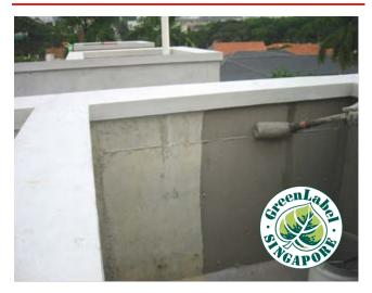
TamSeal 10F is a two-component acrylic modified cementitious coating that requires only on-site mixing to form the ideal product to waterproof and resurface concrete, masonry and most other construction materials. TamSeal 10F provides an effective barrier to waterborne salts and atmospheric gases. It also provides a hardwearing, seamless, waterproof membrane for roofs and concrete protection. TamSeal 10F should not be left unprotected, but covered by tiles or other protective coatings.
